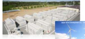
1.5 MW NaS battery alongside 5 MW Solar PV Array, Hokkaido Electric Power Co.
