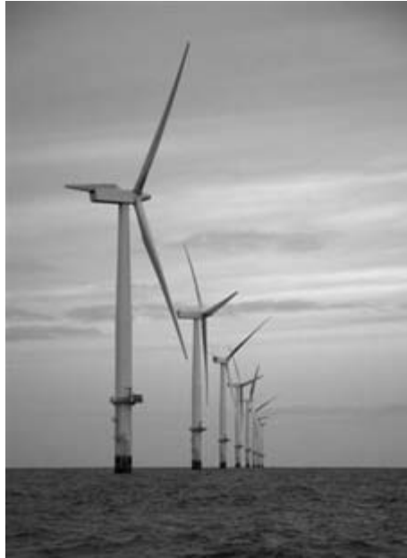
Rhyl Flats Offshore Wind Farm (90 MW) Situated five miles off the North Wales coast, in Liverpool Bay [RWE npower renewables]
