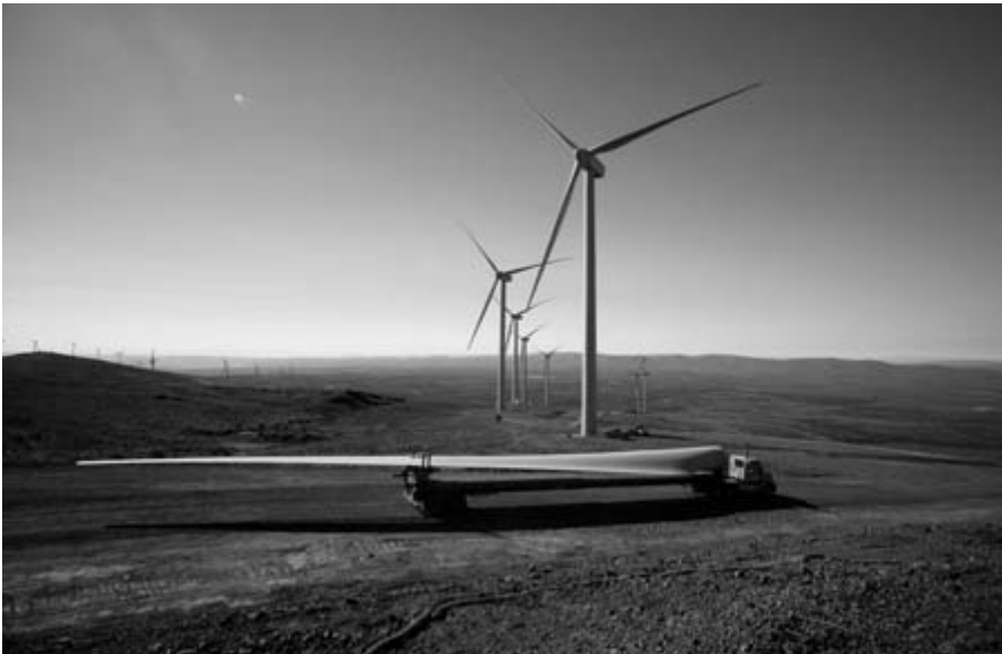
Wild Horse wind farm, Ellensburg, Washington USA (275 MW) Blade delivery. Turbines are 2 MW variable speed using Doubly Fed Induction Generators [RES]
