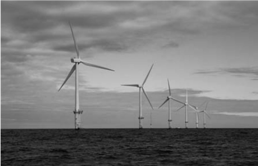
North Hoyle Offshore Wind Farm (60 MW)
