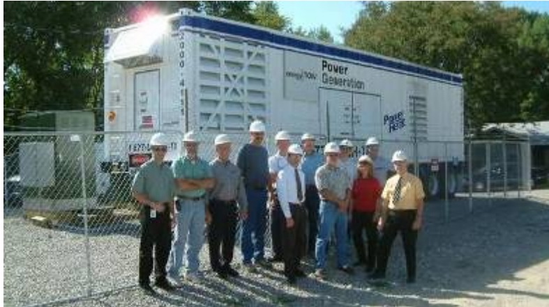
Figure 8-1 Collins Emergency Installation
