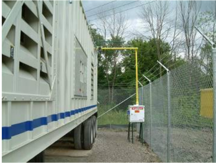
Figure 5-12 Fill Box and Hard Piping to DER
