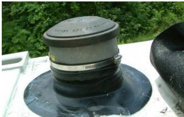
Figure 5-8 Installing External Vent on Generator Shipping Container
