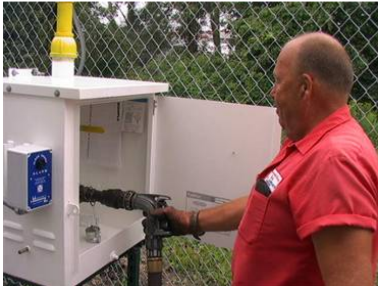
Figure 5-12 Fill Box and Hard Piping to DER
