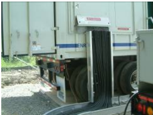
Figure 6-8 Example of Cable Tray for Interconnections
