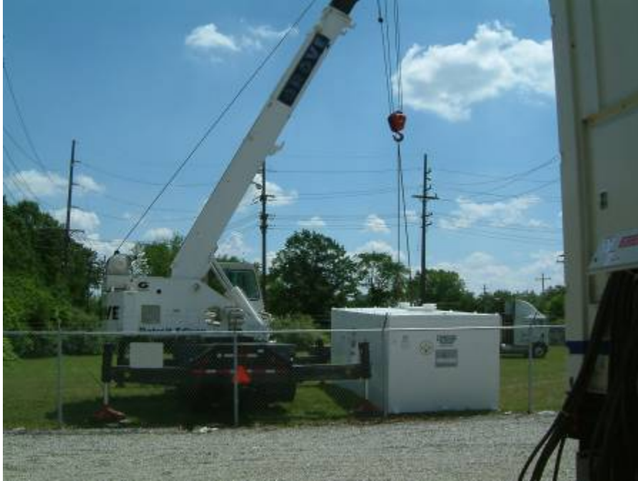
Figure 6-3 Crane Moving External Fuel Tank Into Place
