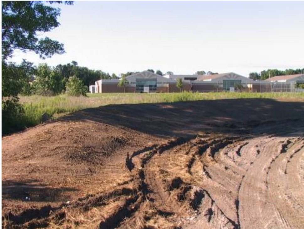
Figure 6-1 Example of Earthen Berm Made of Topsoil From the Site
