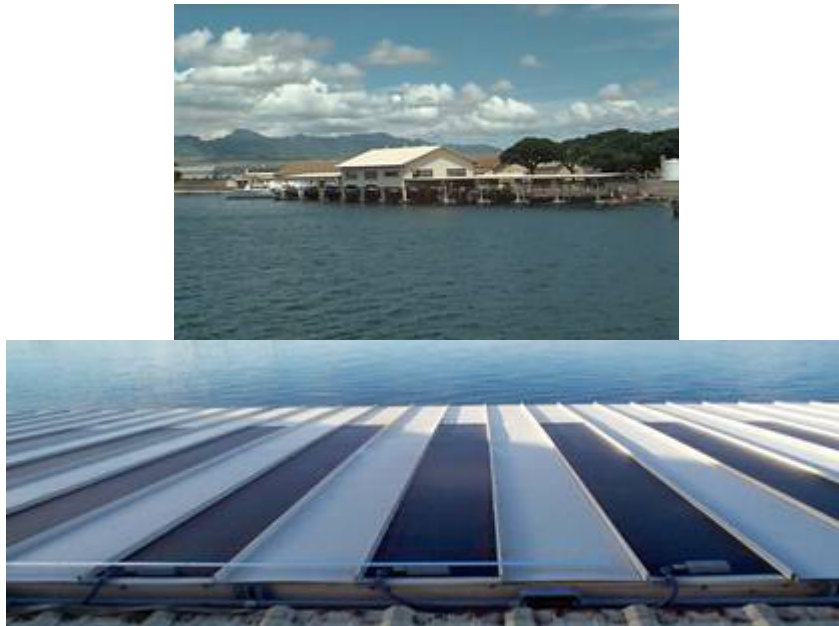
Figure 7-1 Ford Island 2-kW BIPV System – Boat House (top photo) and Standing Seam PV Panels on the Roof (bottom photo)
