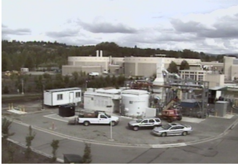
Figure 3-7 1 MW Molten Carbonate fuel cell demonstration unit sited at a Wastewater Treatment Facility in King County, WA. Technology provided by FuelCell Energy
